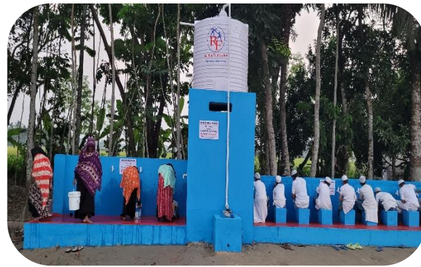
Drinking Water and Wadu Facility in West Bengal
