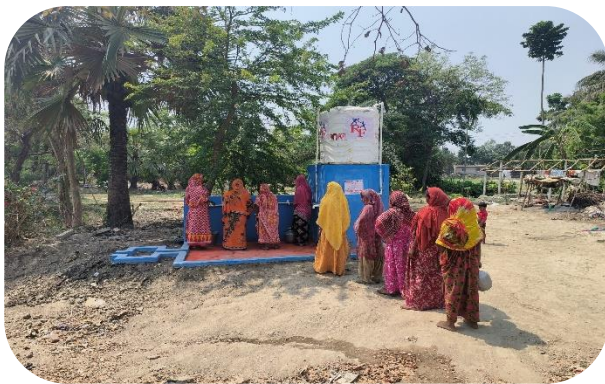
Submersible Water Pump at PargatiChorpara, WB
