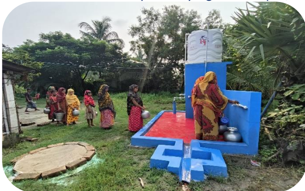
Drinking water pump at Durgamandap North24 PGs, WB
