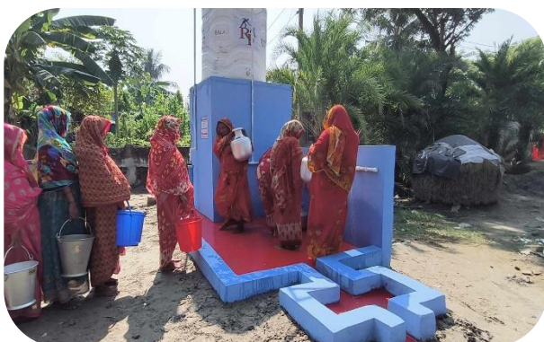
Drinking Water Facility at Goaldah-Minakhan, WB
