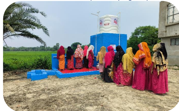
Drinking water pump at Shimulhati, North24 PGs, WB
